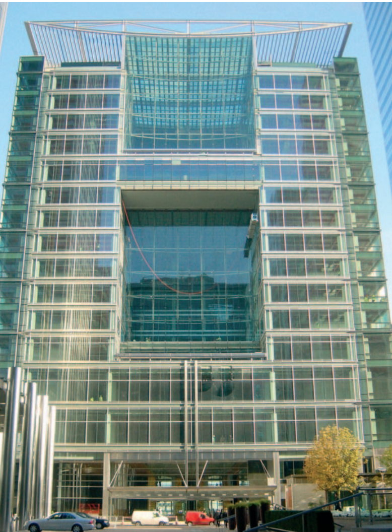
Bank of America Building, 5 Canada Square, Canary Wharf.
