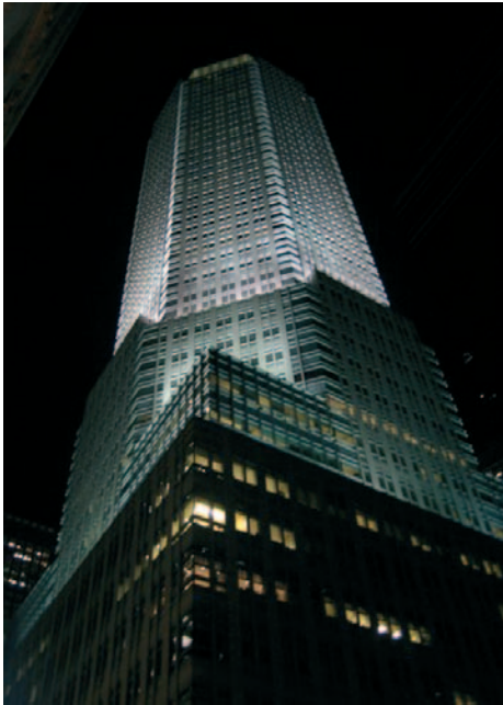
383 Madison Avenue, former Bear Stearns HQ.
